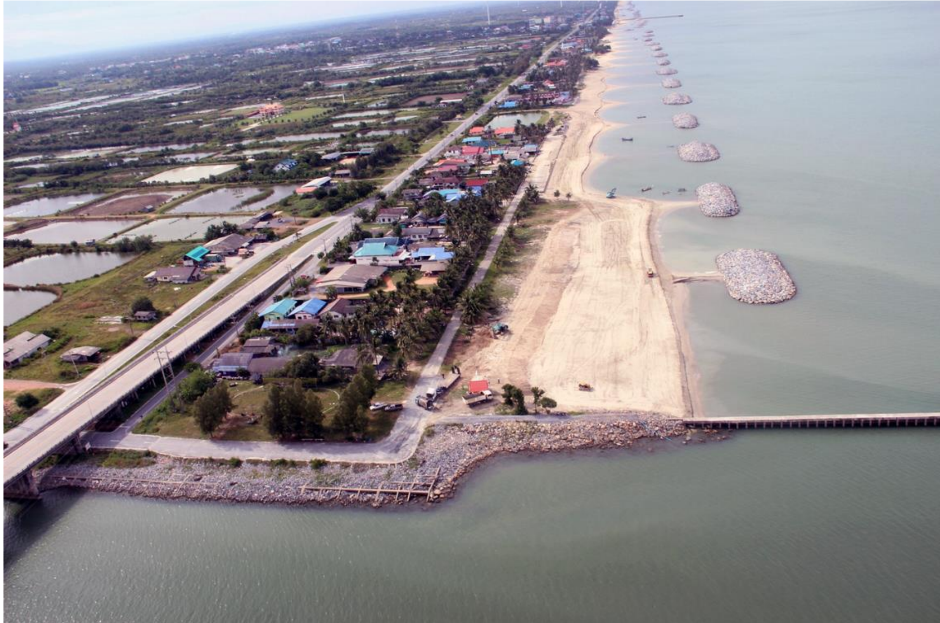
Offshore Breakwater for Coastal Protection in Hua Sai District, Nakornsrihammarat Province
